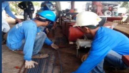
Fabrication of rebar's at fabrication shop for the construction of depot perimeter wall.
